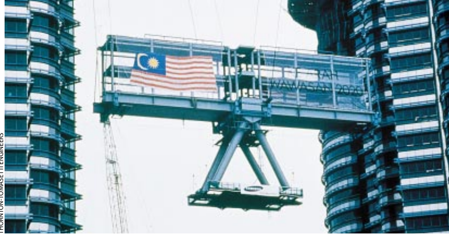
THREE DAYS were needed to lift the 325-metric-ton skybridge after lightning damaged control equipment.
